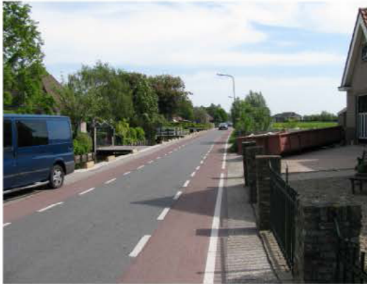
An edge lane road with bicycle priority. Low density suburban/rural area. Roadway used by people cycling and driving. Post speed 35 MPH.
